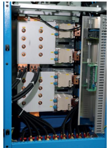
IGBT converter for 3,000 kW
